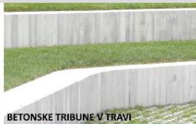
BETONSKE TRIBUNE V TRAVI
